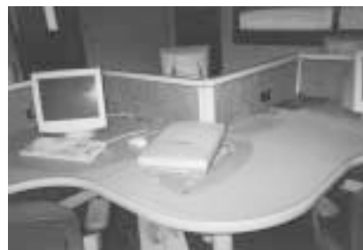
Flood Damaged HIEC Lab
